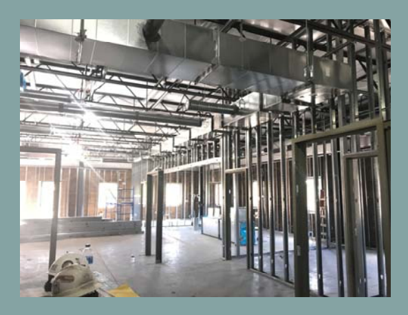
Pic 2: Interior framing for the office area.
